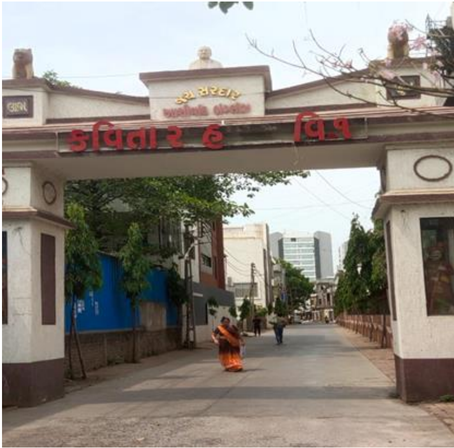
Row House Complex Entrance
